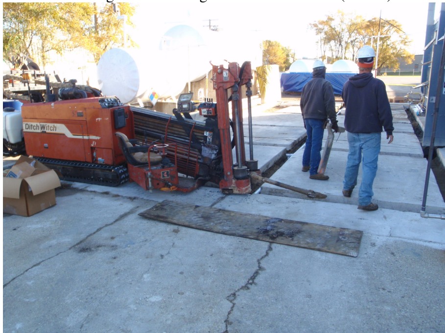
Figure 2. Drilling of Horizontal Wells (Area 1)
