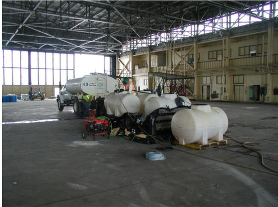
Each well was estimated to have a radius of influence of approximately 10 feet each. Over the course of this project, a total of 75,000 pounds of sodium persulfate and 15,000 pounds of ferrous sulfate were mixed into solution and injected into the groundwater. The injections were completed over a period of 41 days in the field.
