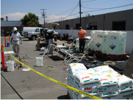
FIGURE 5. Injection of sodium hydroxide solution.
